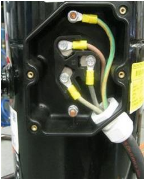
Figure 22: Electrical installation with cable glands, terminal box IP54
